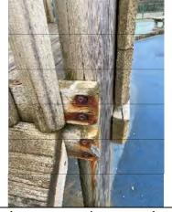
RL Substantial Central bridge structure - Timber elements are starting to rot and fixings have
