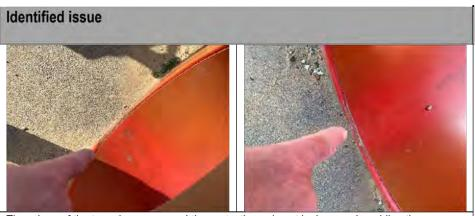
The edges of the tunnel are worn and the protective gel coat is damaged enabling the construction fibre beneath to become exposed with further wear/usage. Replacement or repair needed
